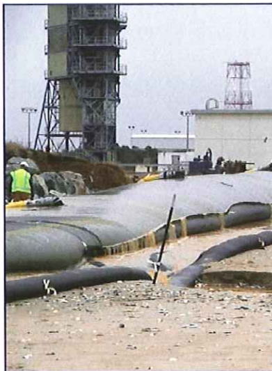
Pump in a pit - Filling Geotubes
