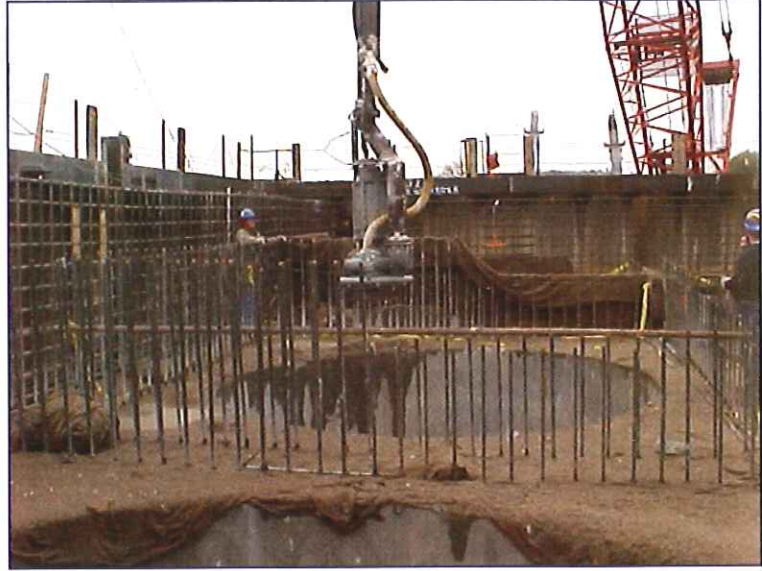
Dredging sand from inside 15 ft. diameter caisson
