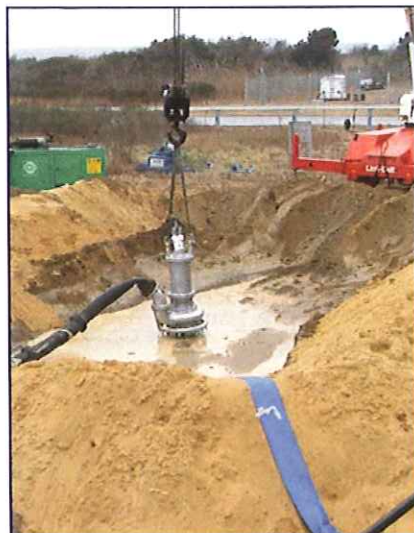
Pump in a pit - Filling Geotubes
