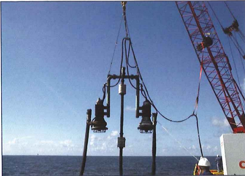
Twin DP-150B's burying pipe offshore
