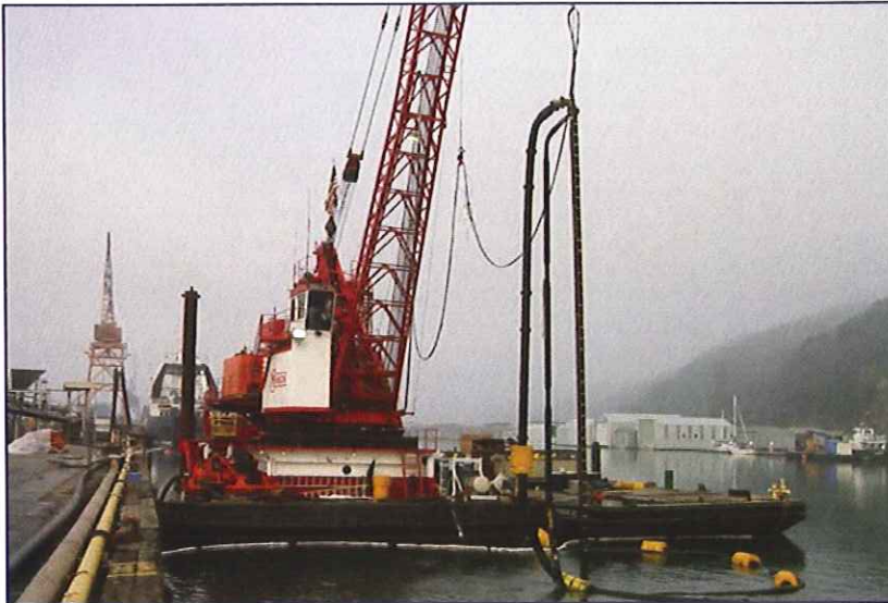
Removing contaminated sediments - very low turbidity
